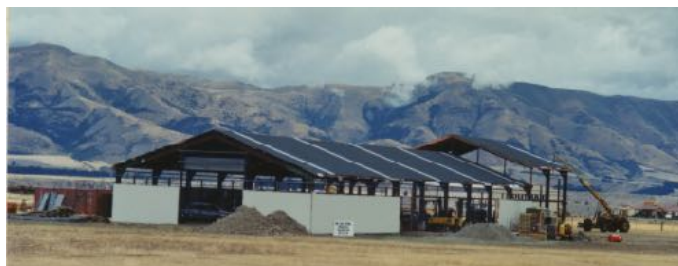
Main building starting to take shape
