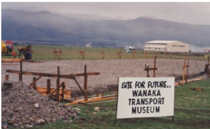
Foundations for 1st Building now known as the Main Building
