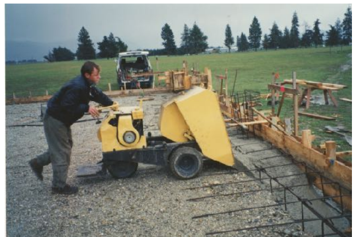
Jason Rhodes working on the concrete foundations of the Main Building
